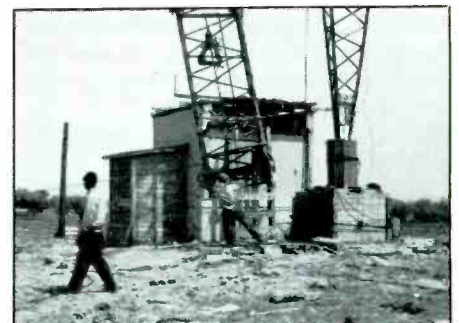
Once the concrete dried, the next section was raised.
