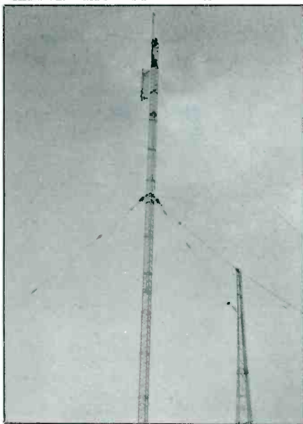
This shot gives a good view of the guy wires.
